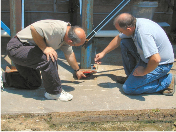
Fig. 3. Load cell installation.
