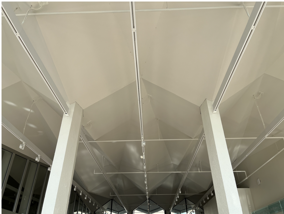
Figure 3.3: The Steinberg ceiling with the mirrors facing downwards.
