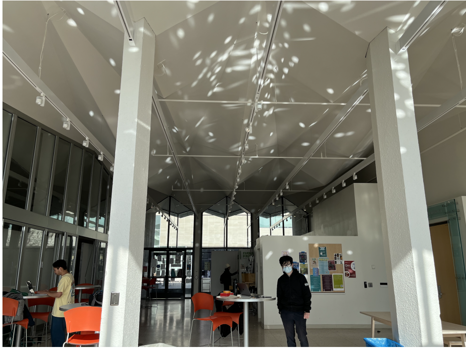
Figure 3.2: The Steinberg ceiling with the mirrors facing upwards.
